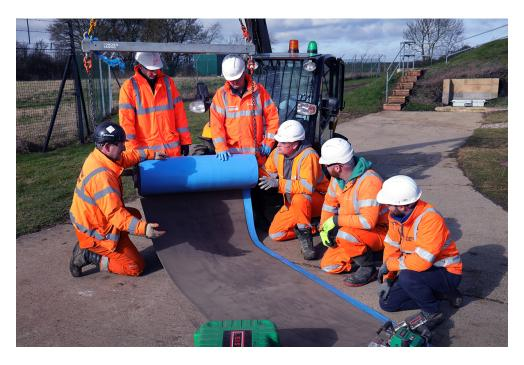
Trialling concrete canvas at our Gazeley Water Treatment Works in Suffolk: this is a much quicker and significantly more carbon-efficient method of laying concrete.
