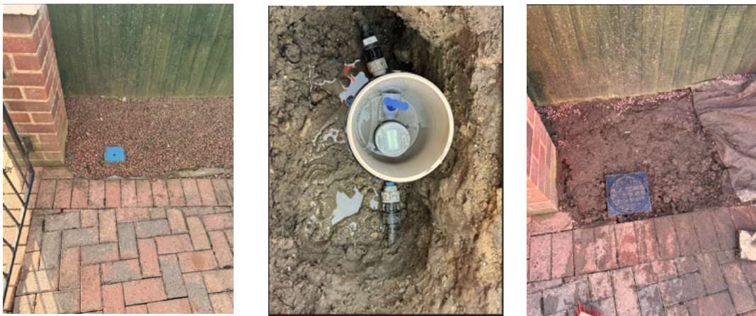
Figure 23: Typical meter replacement (Before, Remove, Replace)
