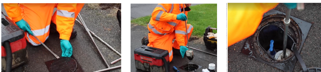
Figure 23: Typical meter replacement (Before, Remove, Replace)
