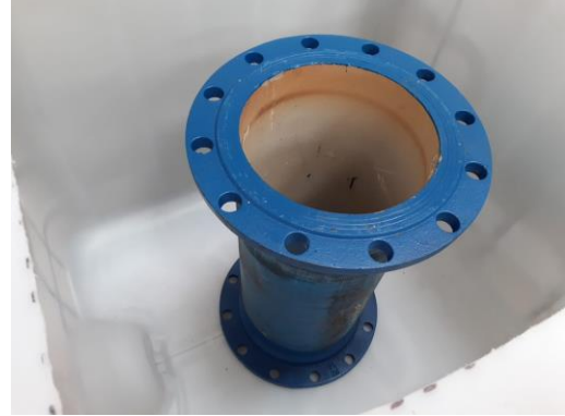
Figure 1 & 2 double flanged ended pipes with 100mm of QD8 coating up the barrel from bottom of pipe standing on the tank floors
