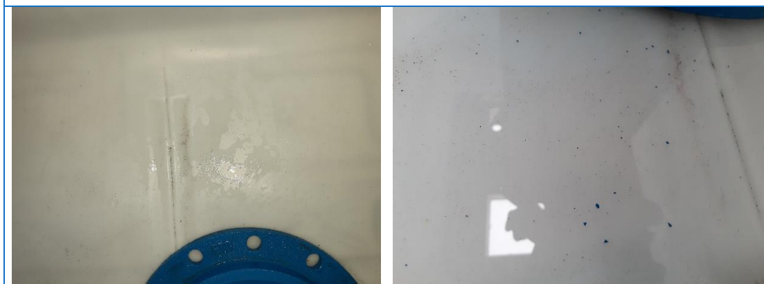
Figure 16 & 17 tank floors looking outside the pipe after tanks drained – some very small flakes of coating visible
