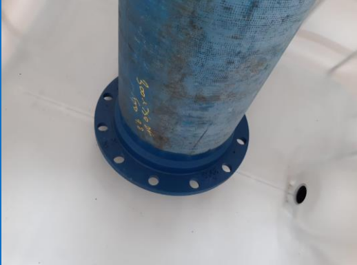
Figure 3 & 4 flanged ends with 100mm of QD8 coating up the barrel from bottom on tank floors
