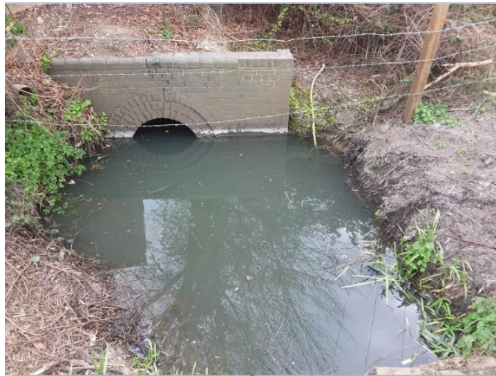
CSO outfall, Offord Cluny Station Lane TPS with water mark clearly demonstrating an almost fully submerged outfall.
