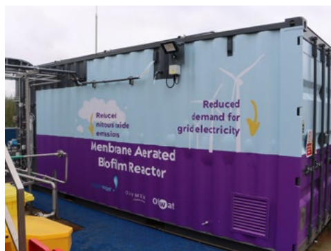
Membrane Aerated Biofilm Reactor at Cambridge
